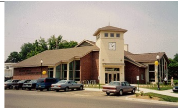
The Kraemer Library & Community Center
